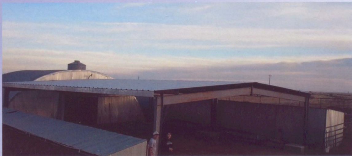
COMPLETE CONSTRUCTION OF THE NEW PAVILION AT THE AG FARM SOUTH OF EADS .
